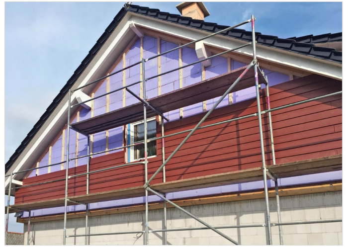
Exterior insulation behind panelling with JACKODUR®
