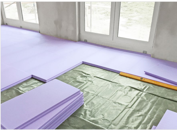
Insulation under screed with JACKODUR®
