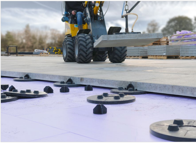
Inverted roof with JACKODUR®
